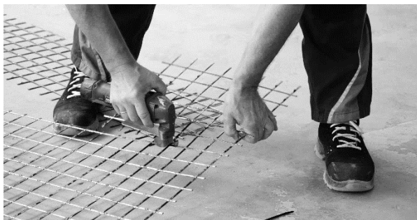
Figure 11: Simple cutting with plate shears
